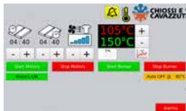
Griff PLC interface
